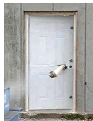
Tornado safe room impact test results: Door assembly failed when perforated
