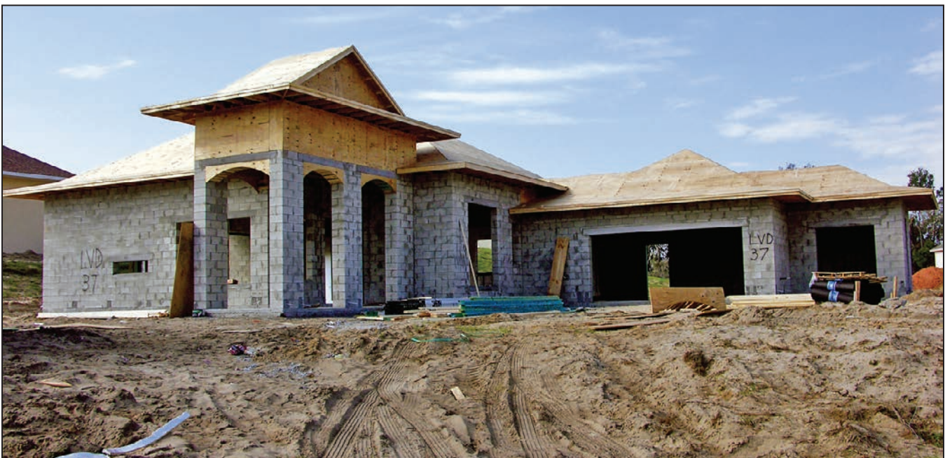
Figure 3-1: Exterior walls constructed of CMUs (New Smyrna Beach, FL, 2007)
